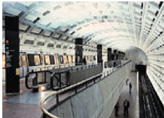
Rosslyn Station, Metrorail
